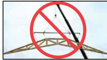
Spreader Bar used is too short for this Truss.
