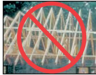
Improper bracing scheme - Continuous TCTLR without Diagonal Bracing
