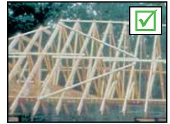
Proper bracing scheme - Continuous TCTLR with Diagonal Bracing.
