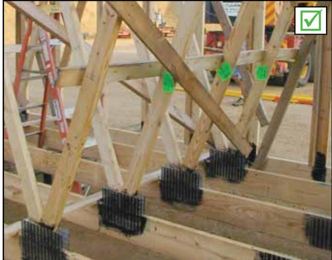
Install Web Member Permanent Lateral Restraint and Diagonal Bracing (or web reinforcement) and Bottom Chord Permanent Lateral Restraint and Diagonal Bracing as required.
